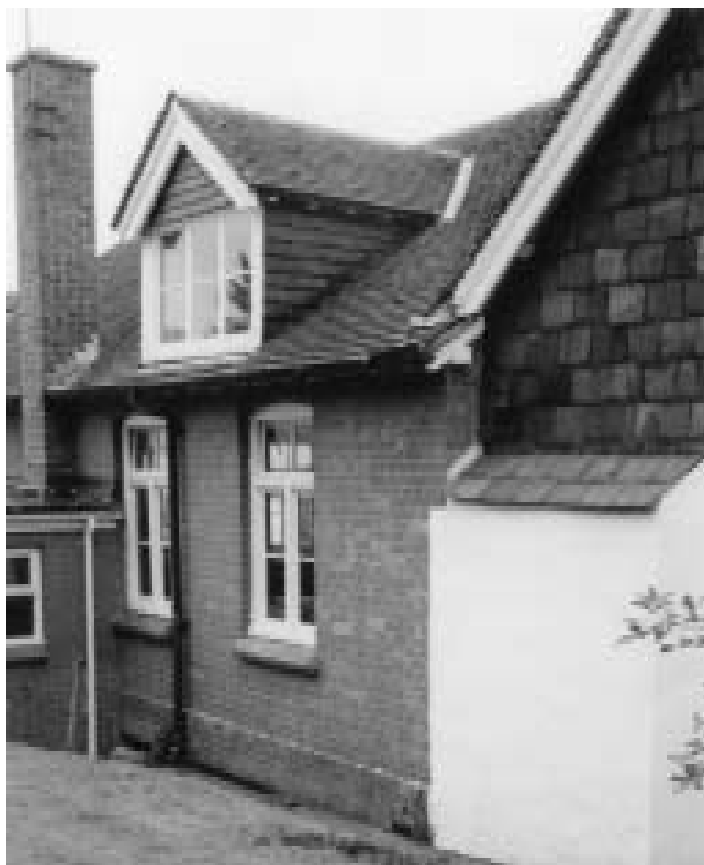
Abbotts Ann Primary School was established in 1831 by Rev. Samuel Best. The brickwork on the left is an original part of the school.
